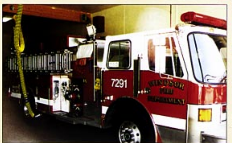
F 42 Extraction for emergency services vehicles.
